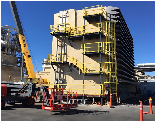
Turbine Intake – Staircase and Ladder.
