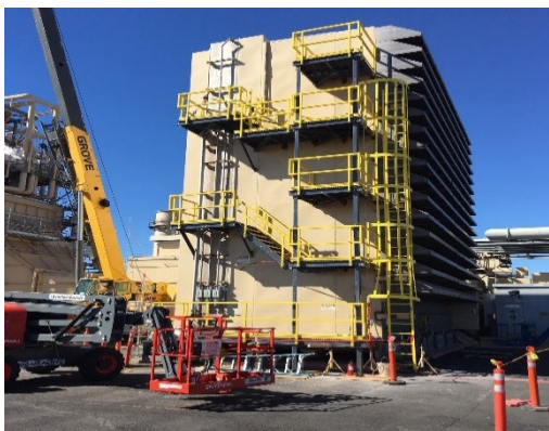
Turbine Intake – Staircase, Ladder, Platform and Handrails (Boulder)
